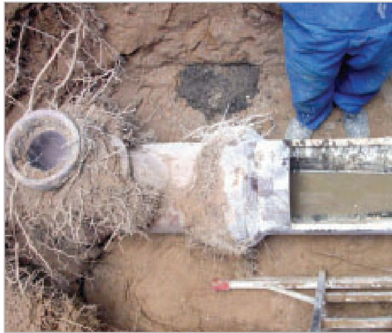
Tree roots are known to invade joints in small diameter wastewater pipelines.
