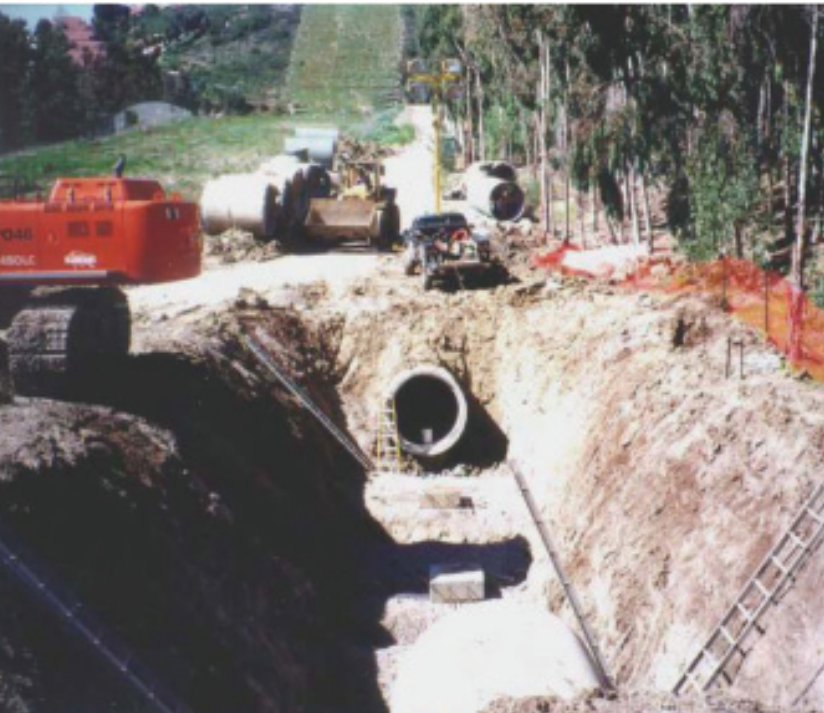
In repairing a large pipeline, extensive excavation may be required.
